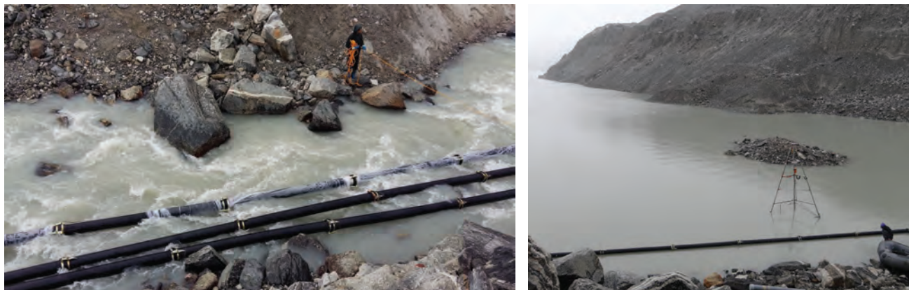
The photos showing the siphoning of South Lhonak Lake for lowering the water level on September 2016
