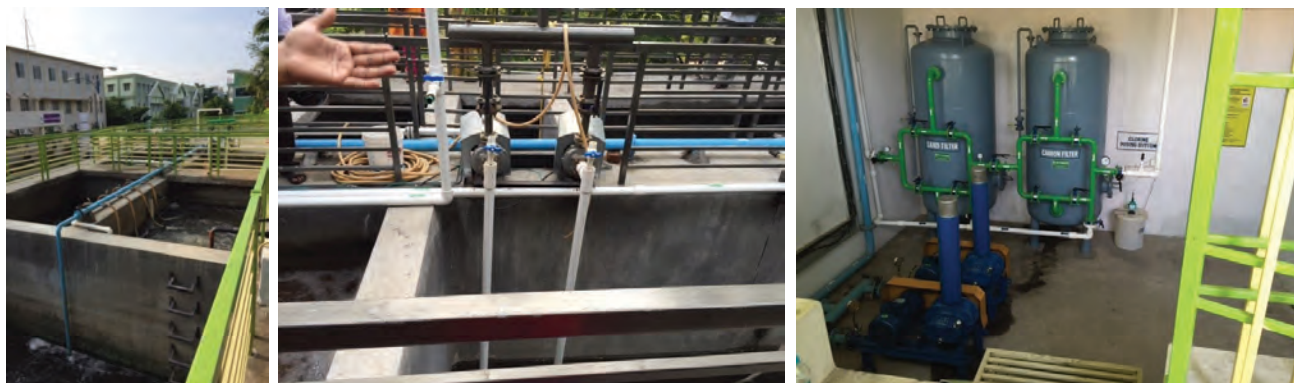
Moving Bed Biofilm Reactor
